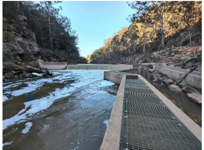
Theresa Park weir and fishway on the Nepean River
