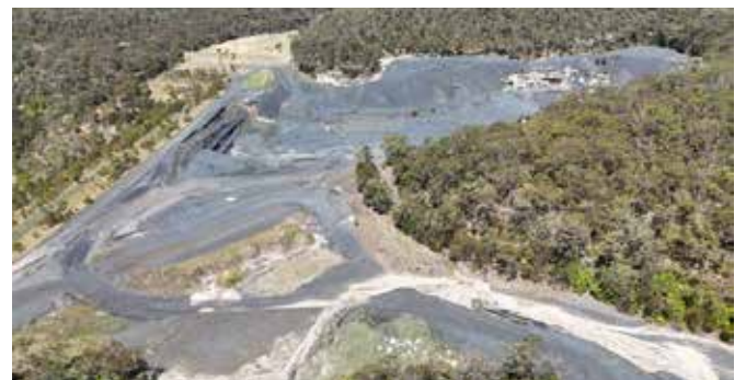
The Western Sydney Pumped Hydro Project by ZEN Energy would utilise a former colliery, in Nattai
