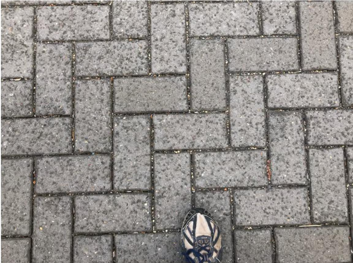
Figure 5.16: A close up view of permeable paving showing closed and open components
