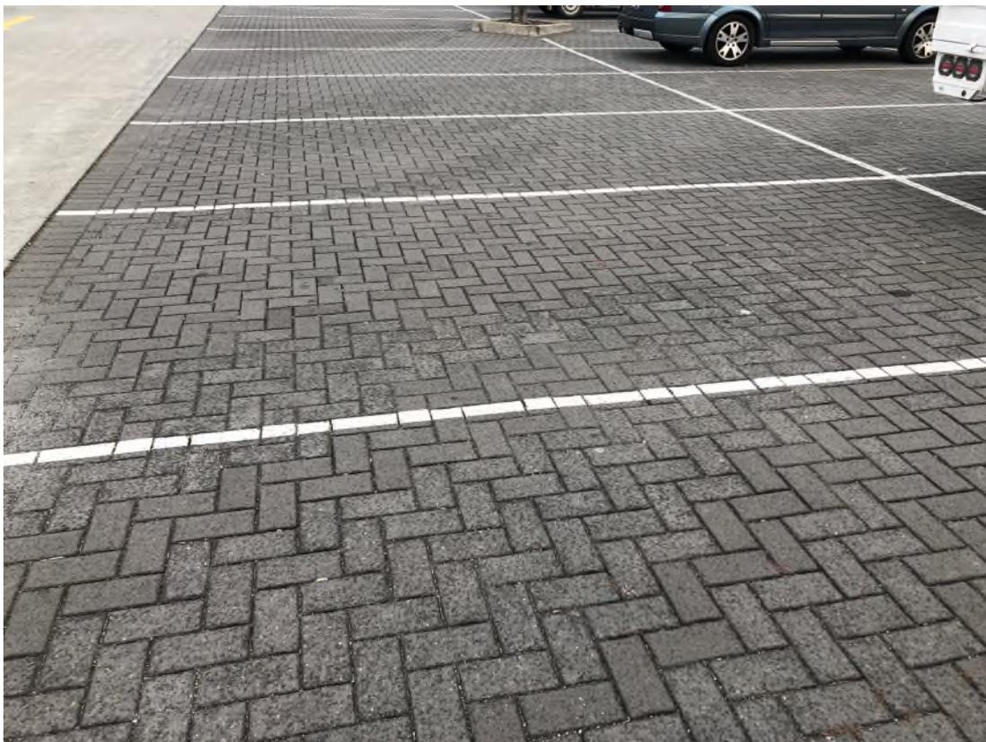
**Figure 5.15: An example of the use of permeable paving in a car park**
