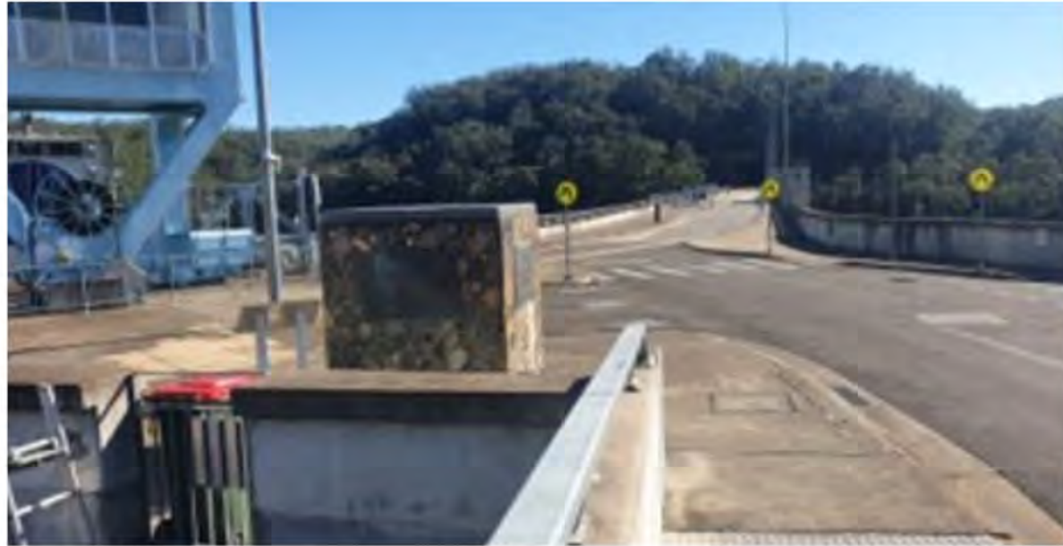
crest (top of the dam wall)
