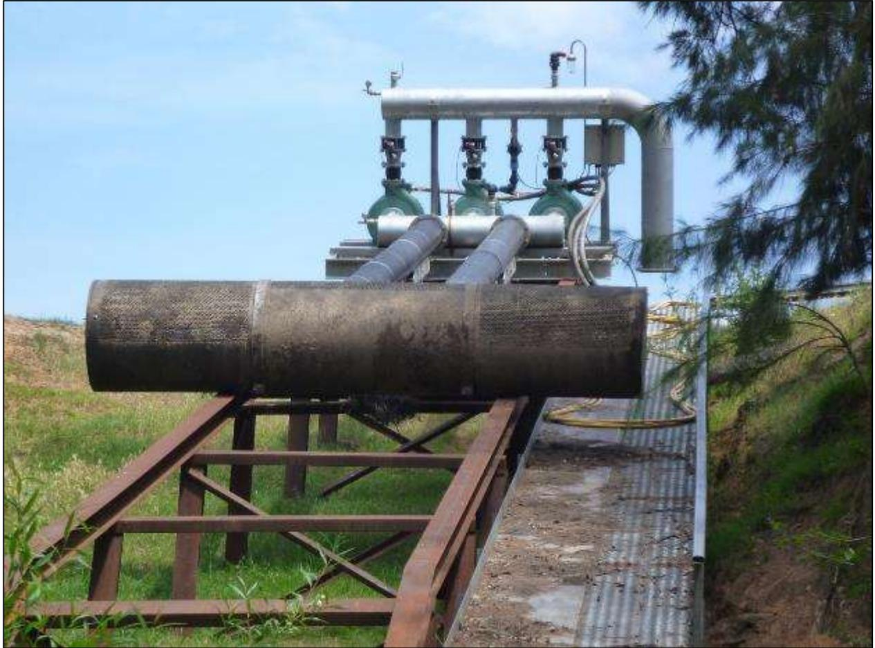
Figure 40. Example of a pump with screen on the Lachlan River
